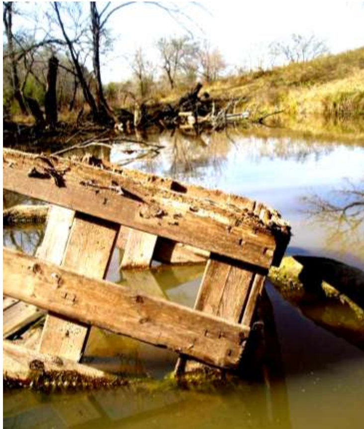
Figure 6.19. Debris at a stream crossing in Caldwell County. Trash is a major issue along stream crossings in rural areas of the watershed.
